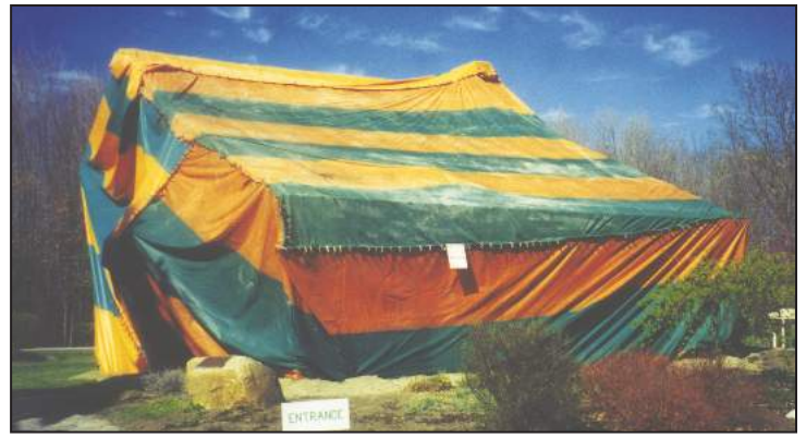
The historic Hartman Log Cabin in Jackson Township had to be tented in the mid-2000s to deal with a powder post beetle infestation.
